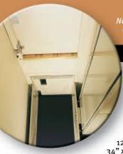
No machine room necessary with the drive system enclosed in the hoistway.
